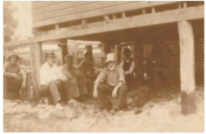
Working-bee volunteers demolishing the old Brunswick church in 1935. Fr McEvoy Parish Priest (back right) can be seen under the building with Bill Peoples, Allan O'Meara, Mr Devine and Mr Reilly.
